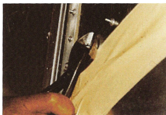
1. PROTRUDING MANDREL IS SNIPPED FLUSH WITH RIVET'S HEAD.
